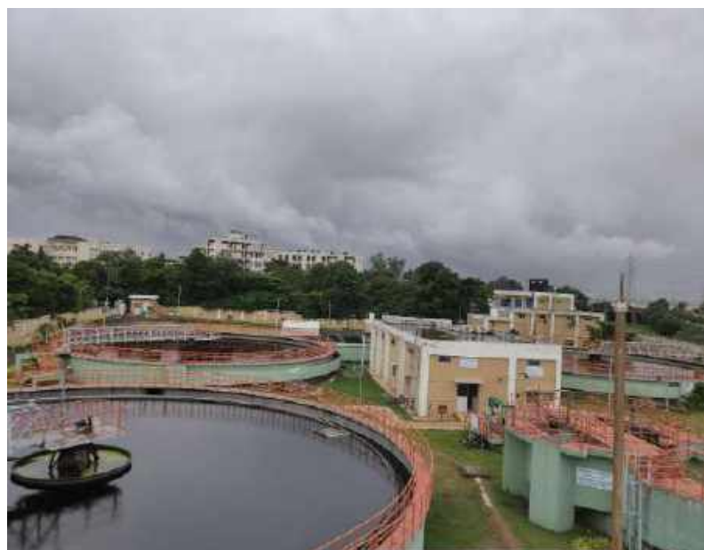
36 MLD STP at CDA-Bidanasi area of Cuttack
