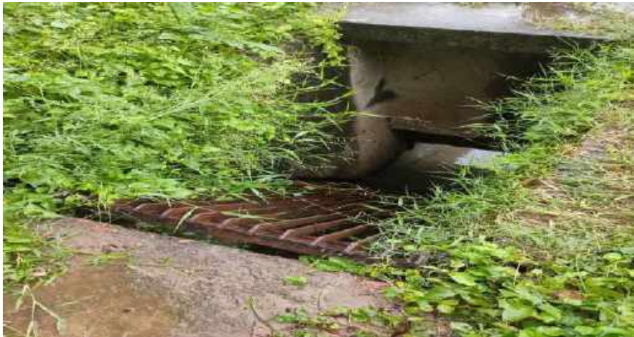
33 MLD STP at Mattagajpur Cuttack
