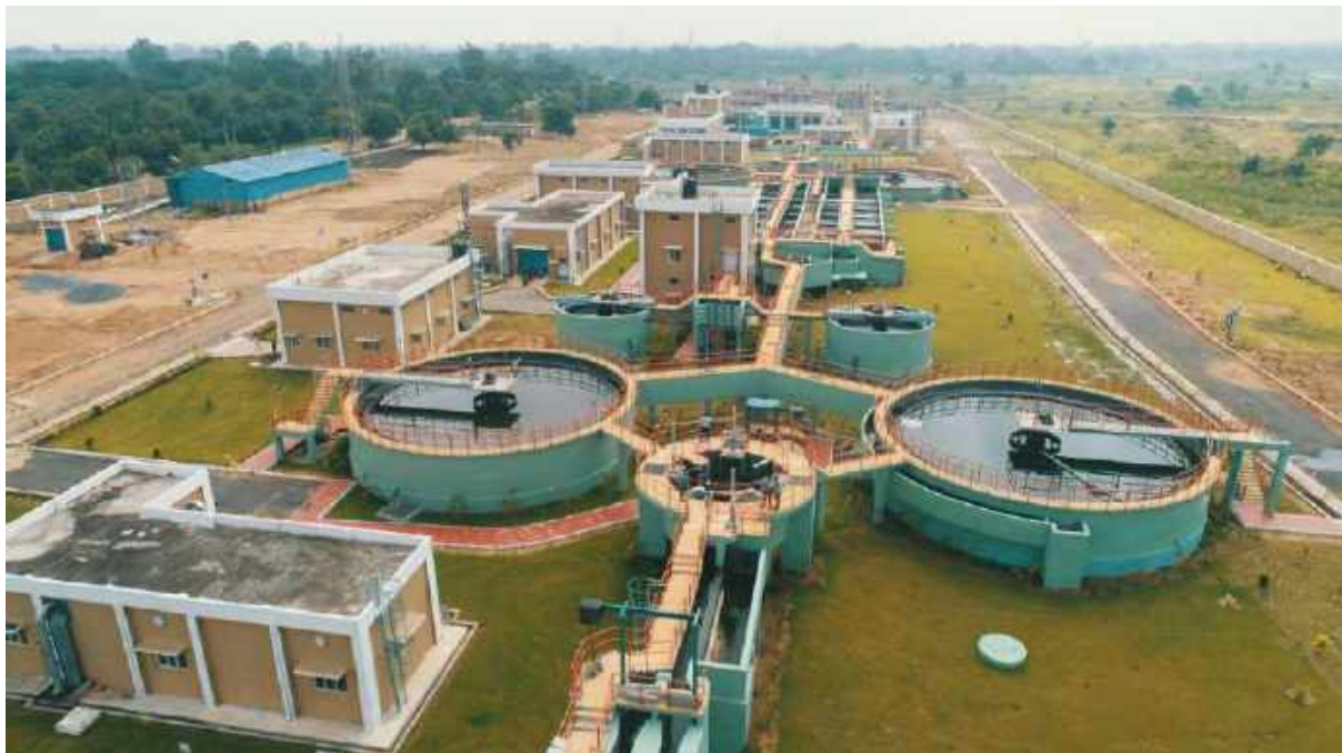
16 MLD STP at Mattagajpur Cuttack
